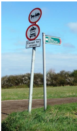
Picture 323. Pole out of correct vertical alignment detracts. Would it be possible to combine all necessary information on one pole?
